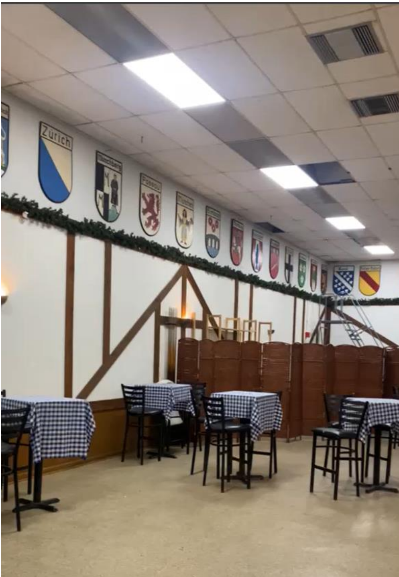
New light fixtures will cut electrical costs by about 50%.
